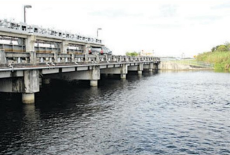
4.73 A weir crosses a drainage canal in the Florida Everglades.
