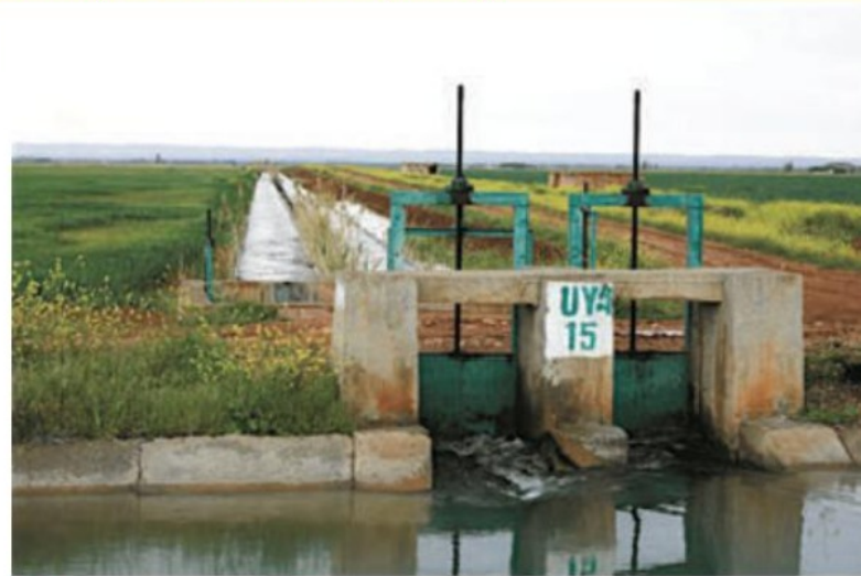
3.85 Sluice gates regulate the flow of water to irrigated fields near Harran, Turkey.
