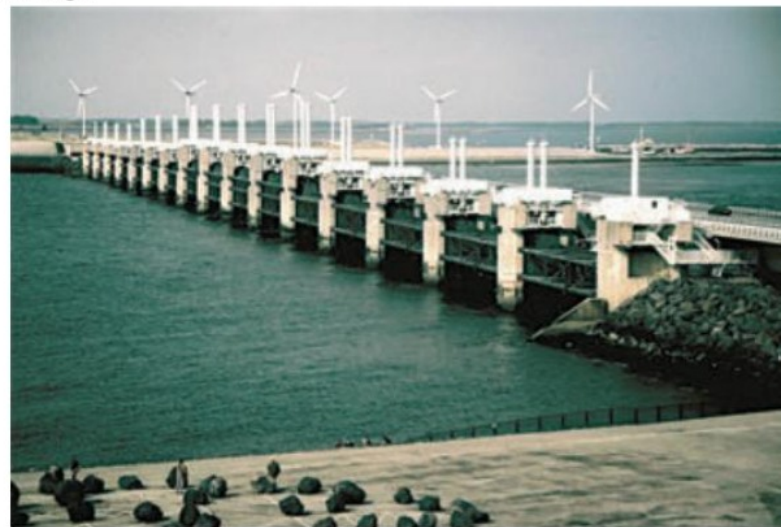
2.43 The world's largest flood barrier is this sluice gate at Neeltje Jans that blocks the inlet of Oosterschelde from the North Sea. Its exposed location makes it ideal for generating electricity using windmills.
