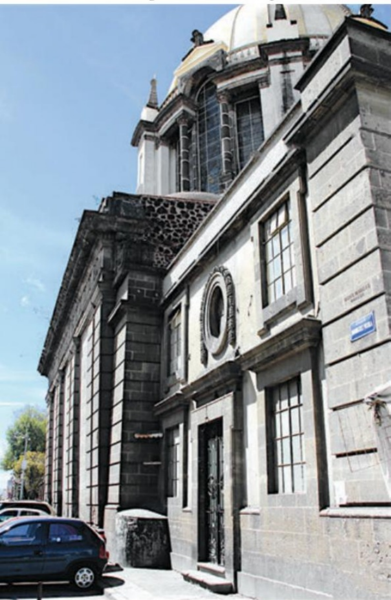
3.39 The Templo de Nuestra Señora de Loreto in Mexico City was completed in 1816. Since that time the facade has been sinking slowly towards the east because of the extraction of groundwater from beneath the building. The effect can be seen here as the walls rise from the pavement at different angles.
