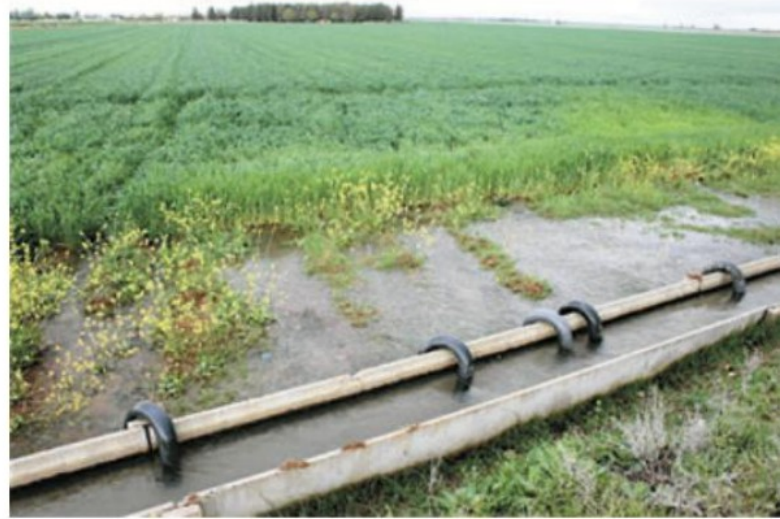
3.82 Drip tubes take water from a distribution canal onto the fields near Harran, Turkey.
