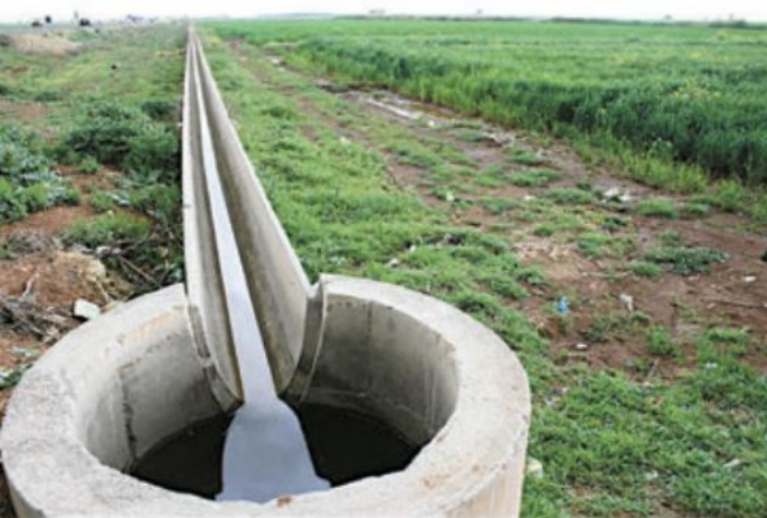
3.81 In the GAP scheme, small distribution canals carry water to individual farms.
