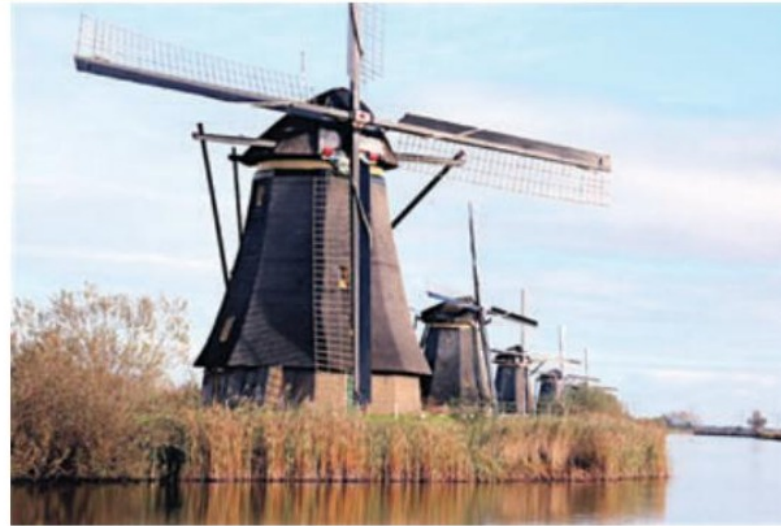
2.36 This windmill at Kinderdijk is one of a series that pumps water to a new level 4.5 metres higher from this polder that lies well below sea level.
