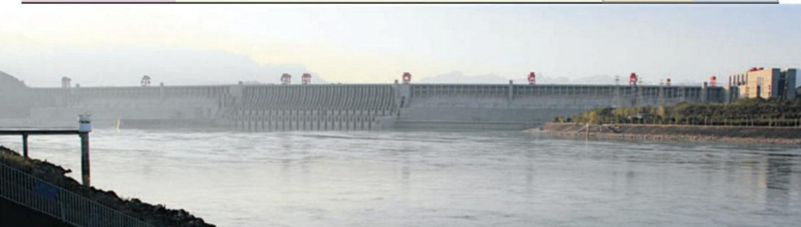
4.25 The main wall of the Three Gorges Dam, showing the spillway in the centre of the wall and four of the hydro-electric plants, two on each side of the spillway.
