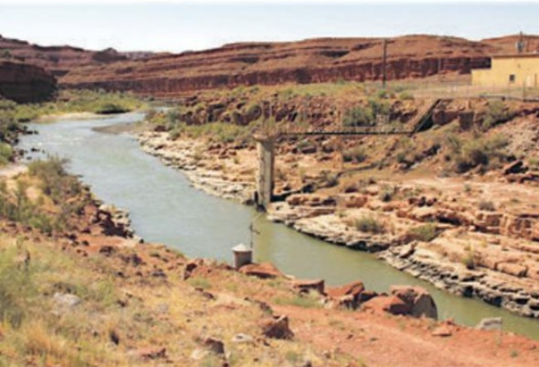
3.21 A stream discharge monitoring station operated by the US Geological Survey as part of the National Streamflow Information Program on the San Juan River, a tributary of the Colorado River, at Bluff, Utah.
