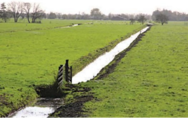
2.40 This polder in Haastrecht is in a peat area and is just over one metre below sea level. Polders in peat areas are larger than elsewhere, and are marked by long, straight drainage channels for flood mitigation.
