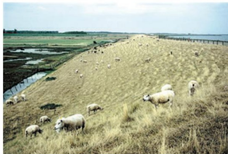
2.33 A section of the coastal dyke near Kouderkerke in Zeeland. The land on the left of the photo is below sea level; the coastal inlet of Oosterschelde is at the right of the photo. Sheep grazing compresses the earth, reducing seepage.
