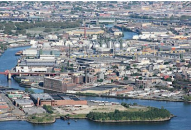
4.9 In stark contrast with the scenes in the previous two photos, the large industrial facility in this photo is the Newtown Creek Wastewater Treatment Plant in Brooklyn, New York, USA. Its eight 42 metre high 'digerger eggs' make it the largest sewage treatment facility operated by the New York City Department of Environmental Protection.
