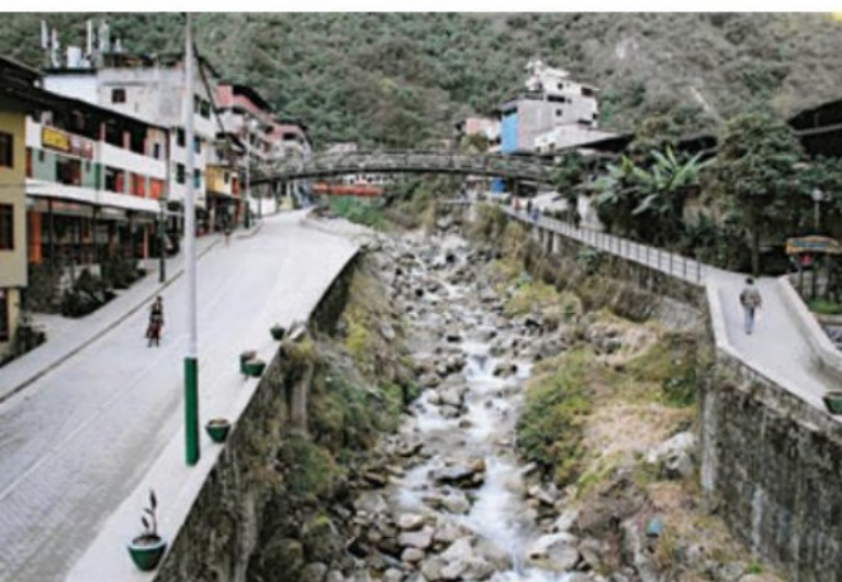
2.9 This canal through the small town of Aguas Calientes, Peru, confines the course of the Rio Alcamayo to a fairly straight tract with high walls to prevent flooding during the spring snow melt in the surrounding Andes Mountains. Straightening the river has raised the rate of discharge, increasing erosion, washing away sediment and leaving only large stones in the stream bed.
