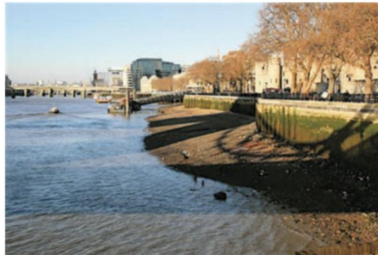
2.21 The embankment along the River Thames in London, UK, was built to prevent flooding, and has been raised several times as the land has subsided and the flood threat has increased.
