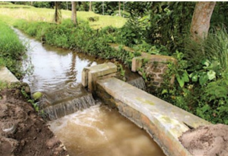
3.33 The network of irrigation channels in Bali is complex and well established. In this view, water from a single canal in Bangkiang Sidem is diverted into several different farms in measured proportions according to the widths of the channels.
