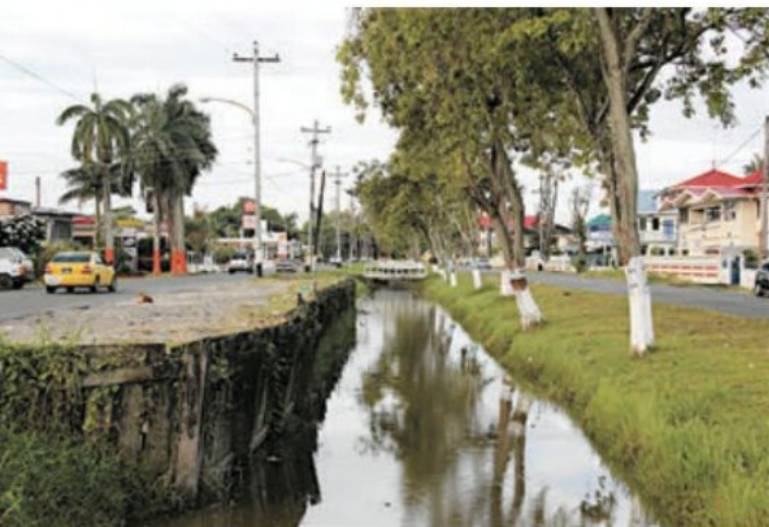
2.20 Guyana's capital city, Georgetown, is flat, low-lying and flood-prone. The city's natural streamflow has been diverted through a network of canals to relieve the threat of flooding.
