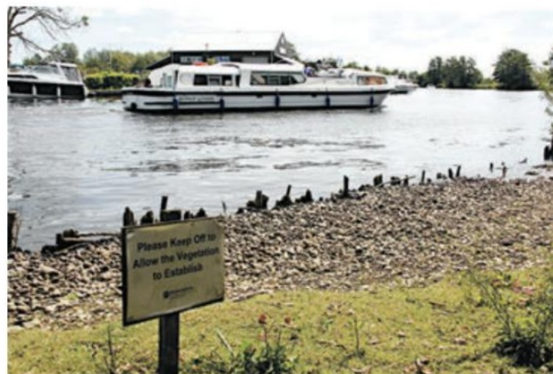
4.47 An area of bank re-stabilisation has been established in an attempt to restore the damage from erosion by boat wake.
