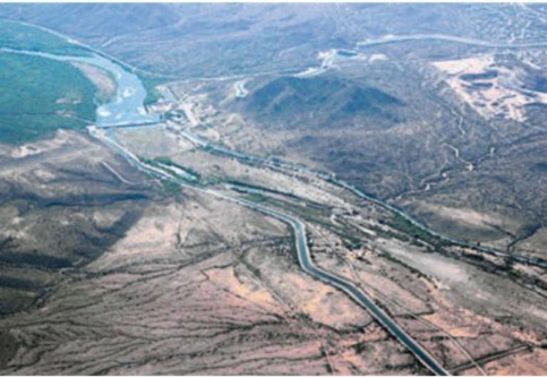
2.15 In addition to flood mitigation, this small dam on the Salt River, north-east of Phoenix, Arizona, USA, serves to distribute water for irrigation during the periods between floods.
