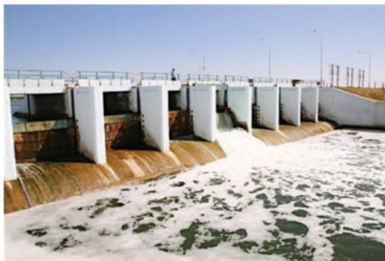
3.66 The weir in the Kokaral Dam helps manage the water level of the northern Aral Sea, which is rising once again.
