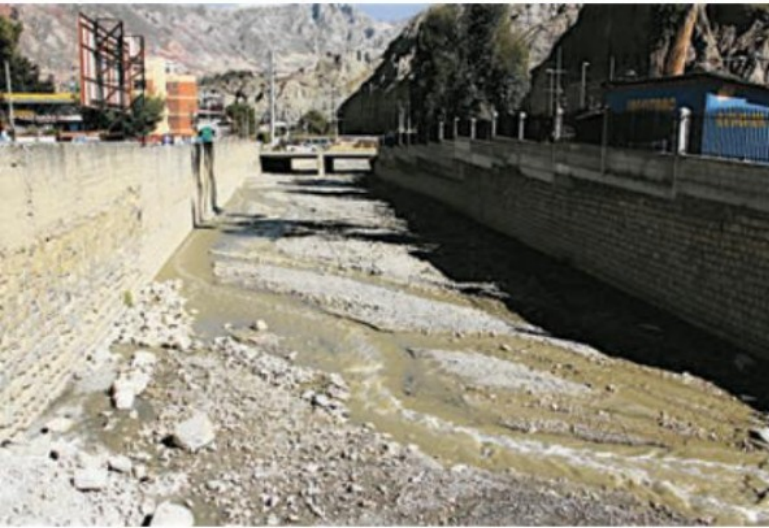
2.18 A small tributary of the Río Choqueyapu in La Paz, Bolivia, has been canalised, straightening and deepening the natural stream channel.
