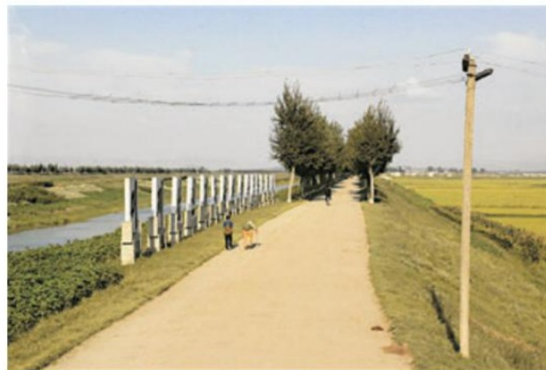
2.17 An artificial levee protects this area of rice farming near Sinchon in North Korea. The irrigation canal that has been built on the levee carries water at a higher level than the surrounding farmland.
