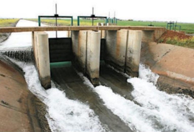
3.80 Sluice gates regulate the flow of water through the canals of the GAP scheme according to need.
