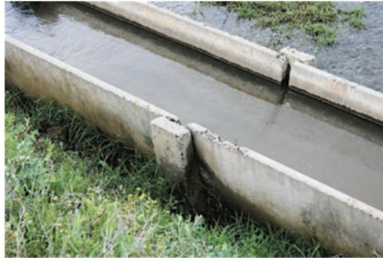
3.91 A distribution canal near Harran, Turkey, leaks water through the joint between concrete sections. Water losses are significant due to leaks, seepage and evaporation.
