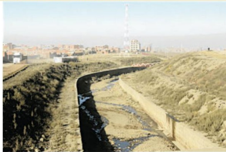
2.10 This canal in El Alto, Bolivia, has sides that force the stream within it to meander within the confines of the canal walls.
